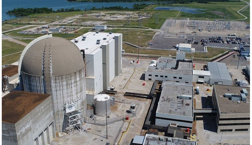
Wolf Creek Nuclear Generating Station lies at one end of the Wolf Creek-Blackberry project. | Office of Nuclear Energy
